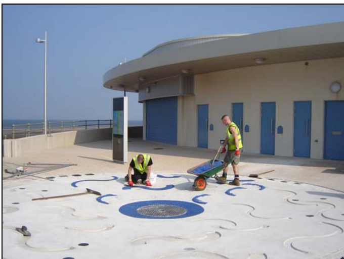
Installation of resin bound glass to the water feature.
