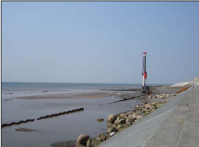
Piling works continue on the beach
