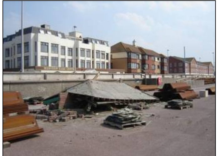
Demolition of promenade shelters
