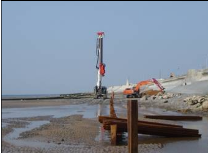
Piling works have begun on Cleveleys beach
