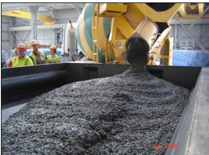
Casting a stepped revetment unit
