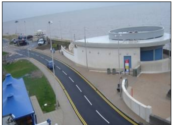
Aerial view of north end of the site
