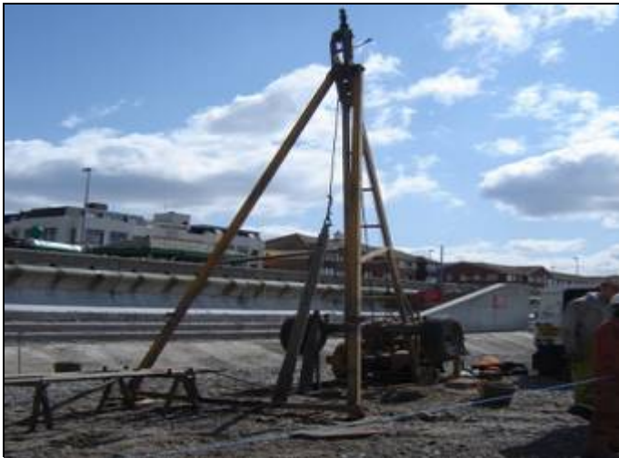
Drilling boreholes for Phase 4 works
