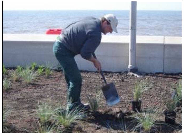
Landscaping works in progress
