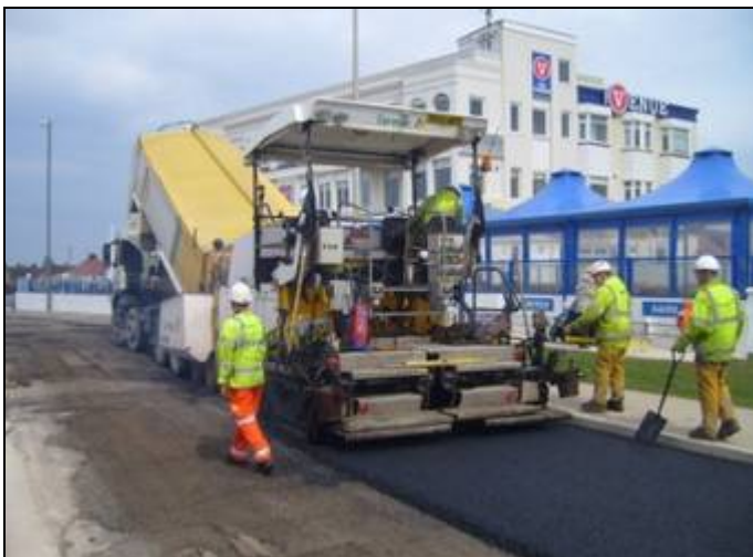
Placing new road surface to north of site
