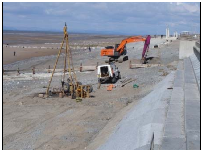
Boreholes being taken on Cleveleys beach
