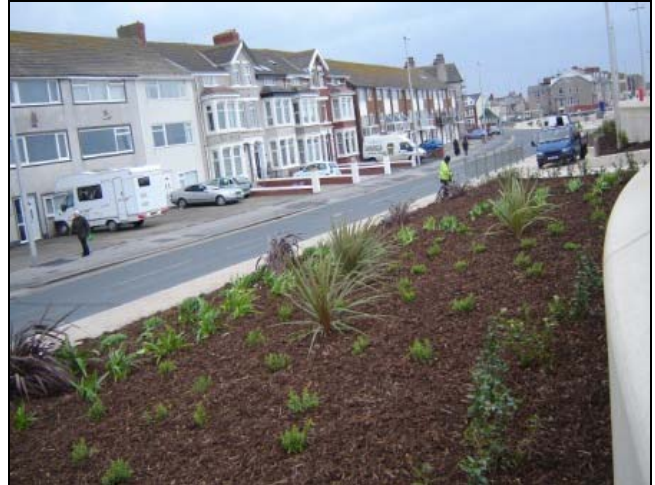
Landscaping works have been completed
