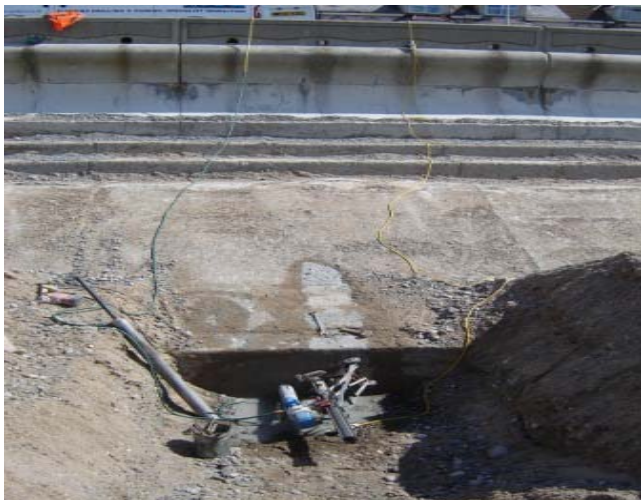
Core samples being taken from the existing defences
