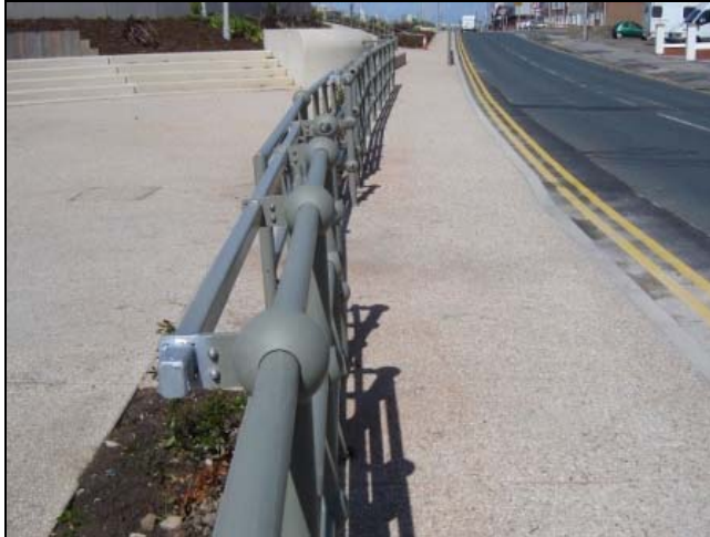
New fencing has been installed
