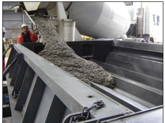
Precasting of the concrete units has already begun
