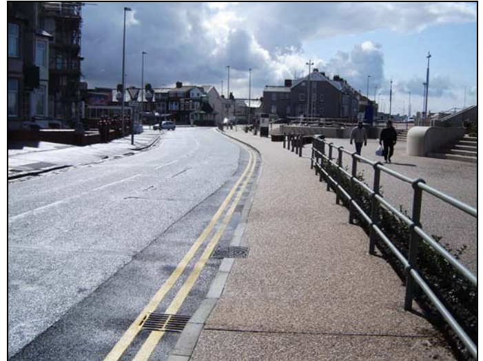
The road on North Promenade has now been re-lined
