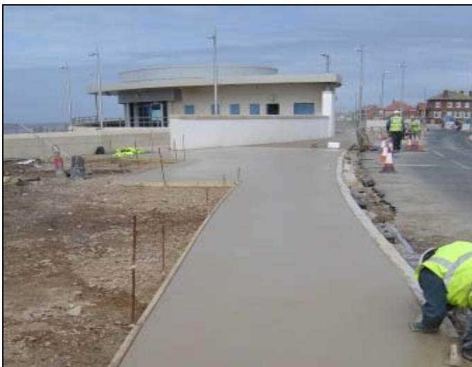
Construction of the roadside footpath in progress
