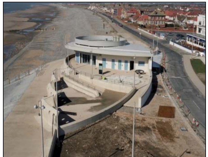
The new café building forms the focal point to the north of the site
