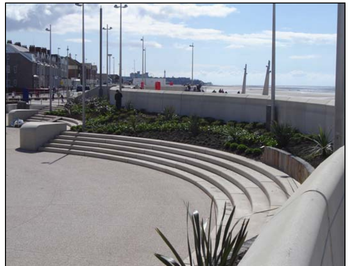
Landscaping works have begun to the new works
