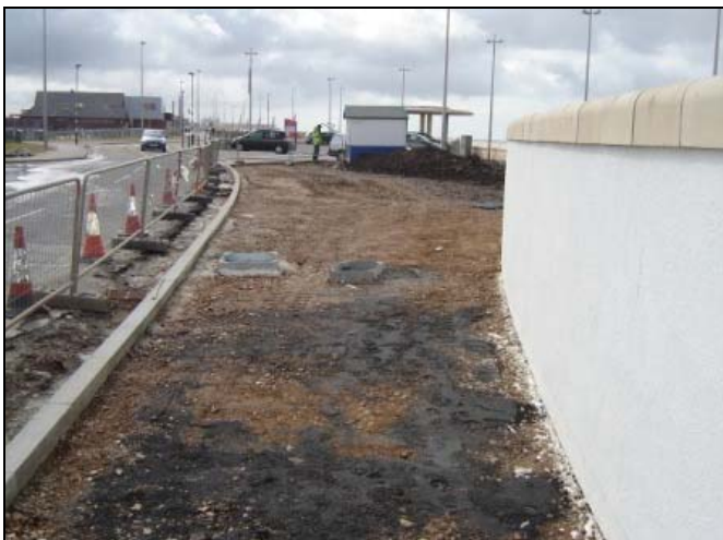
The northern roadside kerbing has been prepared for concreting
