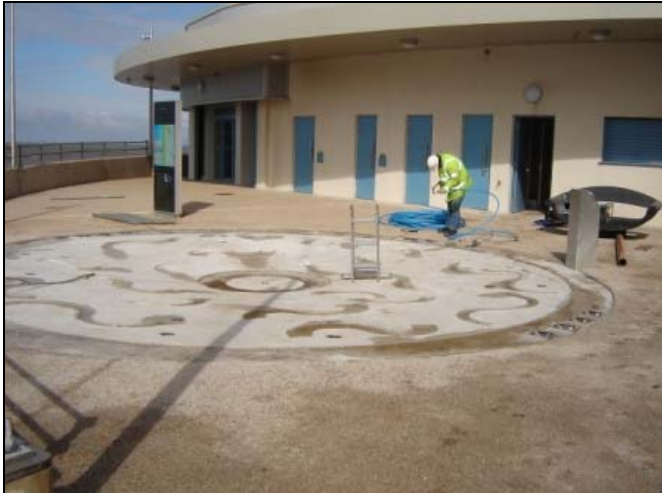
Work on the new interactive water feature is almost complete
