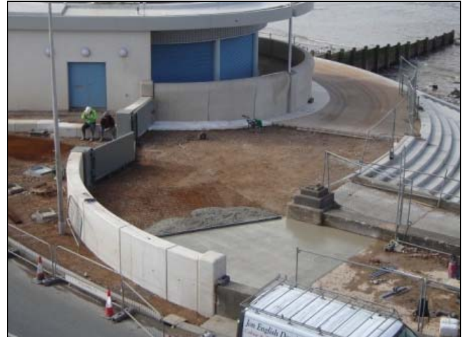
Concreting the new promenade tie-in to the north of the site
