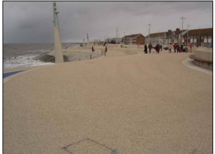
The new promenade works
