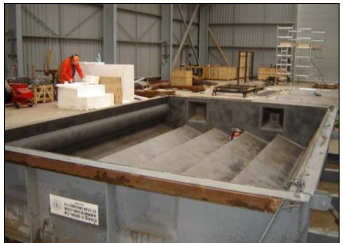
The SLP precast yard on the former ICI site in Thornton
