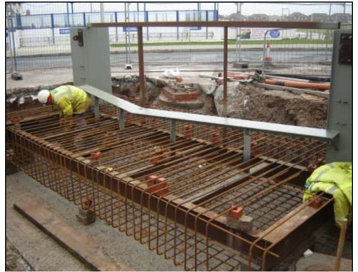
Construction of the north stormgate base
