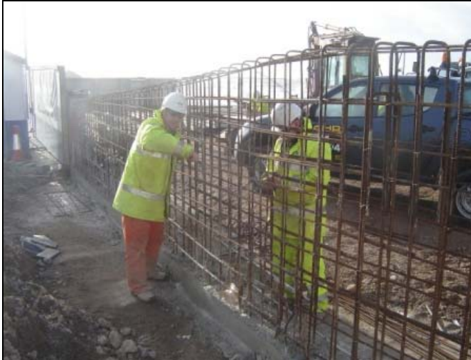
Construction of steel reinforcement cage for rear wall tie-in
