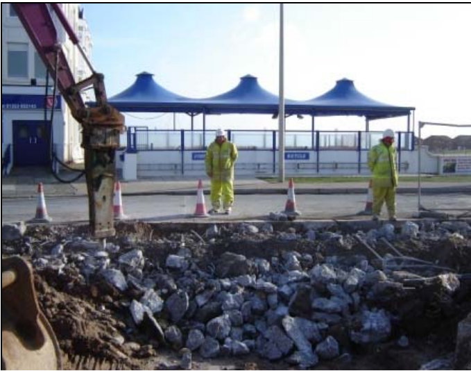
Demolition of the existing promenade
