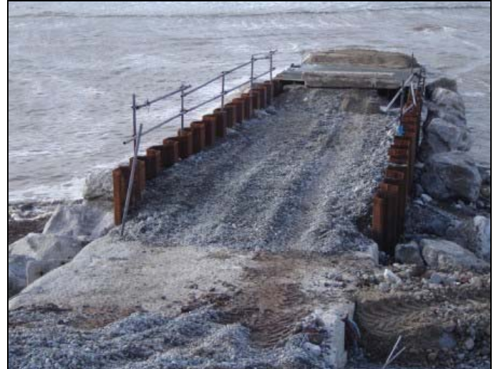
Concreting of slade extension
