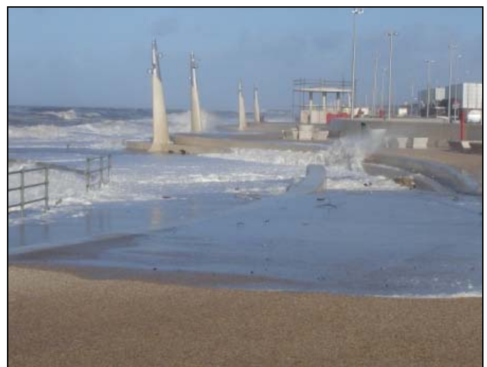
While spray covered the lower deck, the upper deck of the defences was largely untouched
