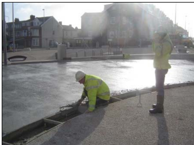
Concreting works to the plaza area
