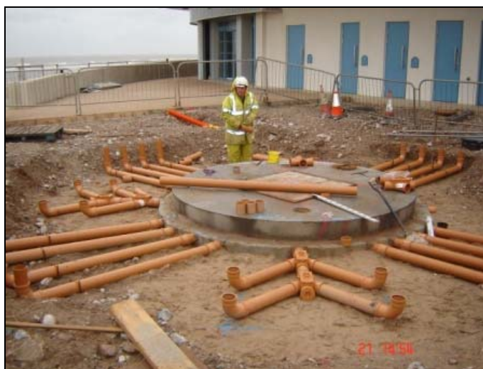
Installation of the pipework for the interactive water jets
