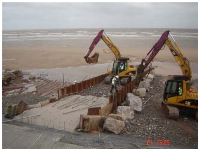
Construction of the new slade extension in progress
