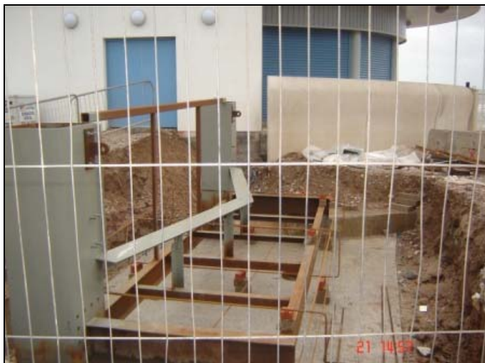
Installing the storm gate adjacent to the café building
