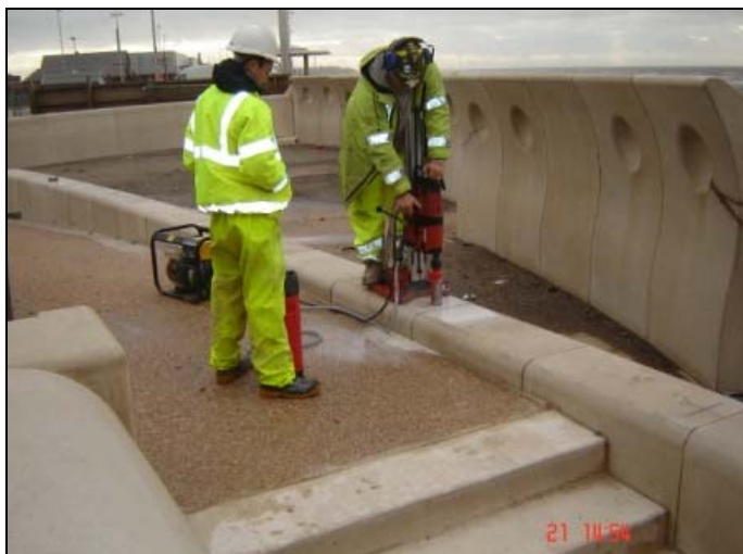
Coring the concrete wall for installation of handrailing
