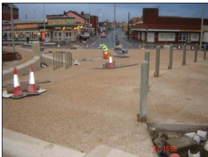
Installation of bollards, cycle racks and seating
