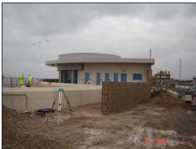
Construction of the café access has continued
