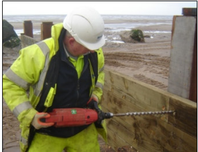
Fixing new groyne timbers
