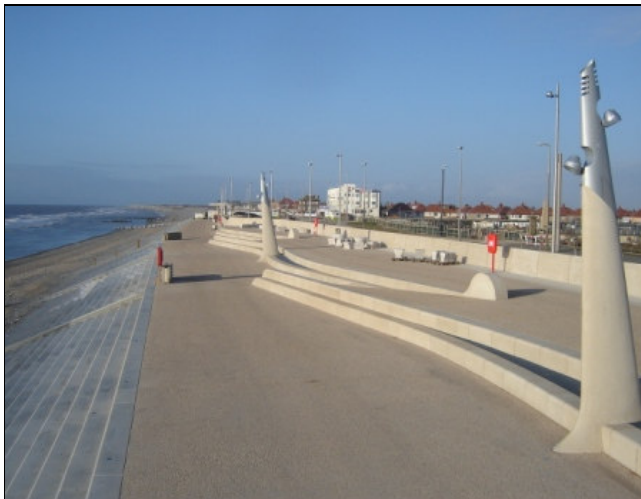
Phase 2 of the works has been nominated for a top ICE North-West award
