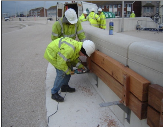
Fixing timber seating on promenade
