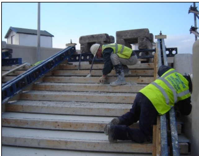
Construction of the southern plaza steps
