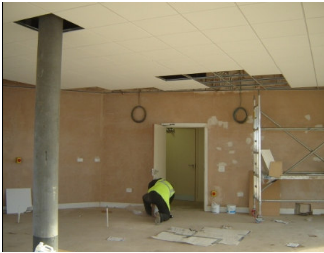
Painting works in the main café area
