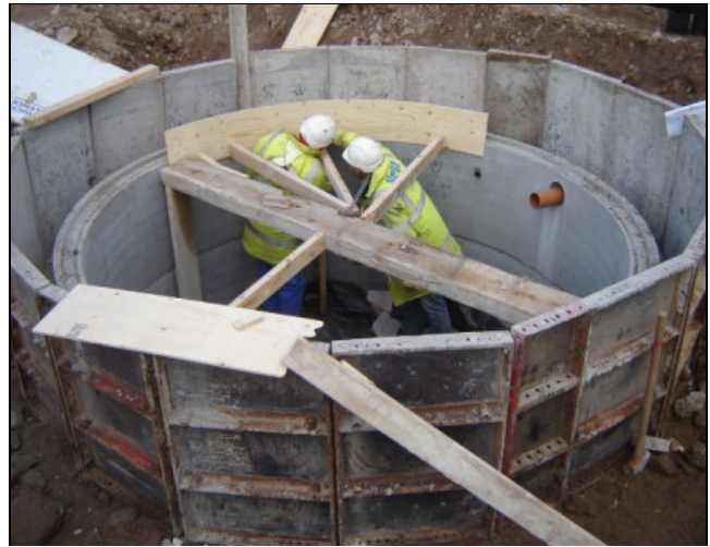
Construction of the interactive water feature
