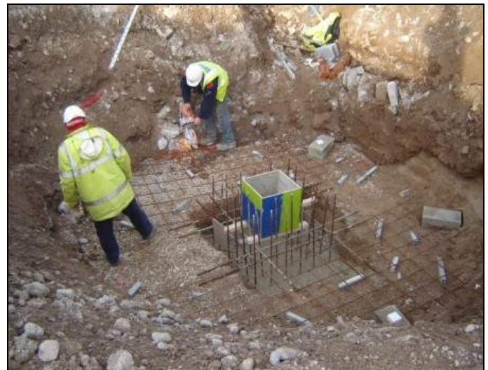
Construction of the water feature has begun
