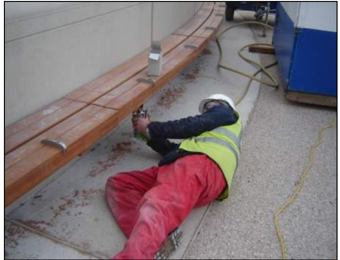
Installing seating along new promenade
