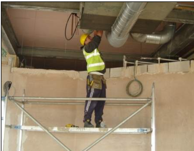
Fitting out of the new café building
