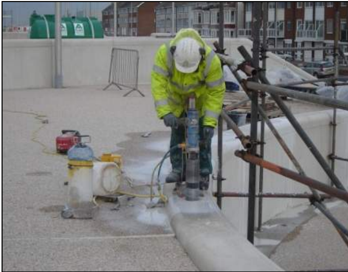
Coring plaza wall for installing recessed lighting
