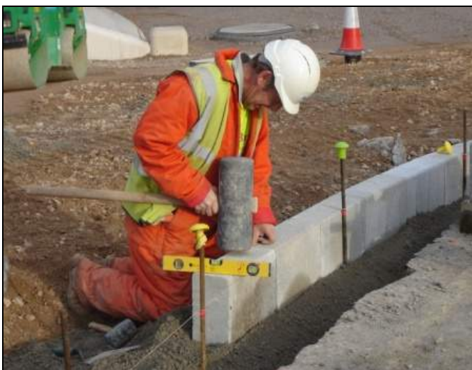
Laying kerbs alongside North Promenade
