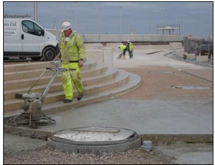
Concreting works around the plaza area
