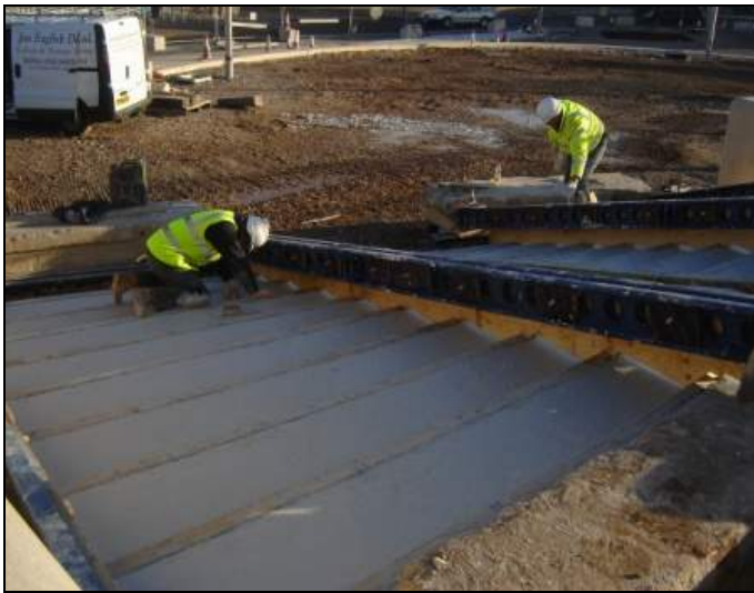
Construction of the plaza steps in progress
