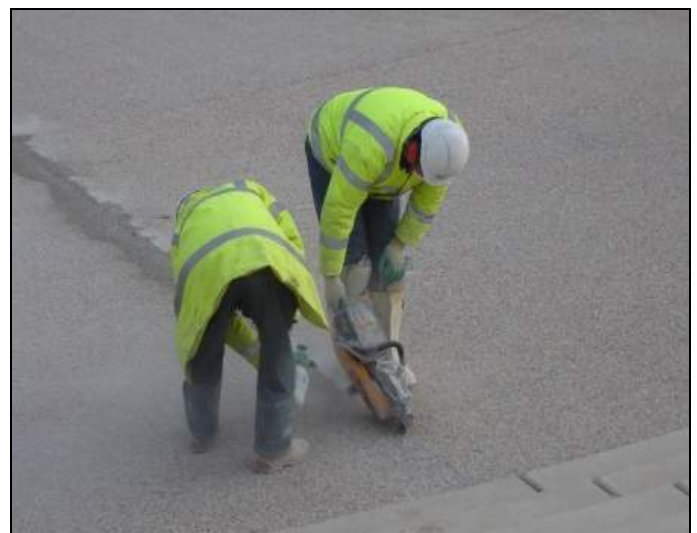
Cutting construction joints in the plaza area
