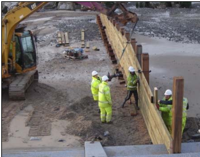
Construction of a timber groyne in progress
