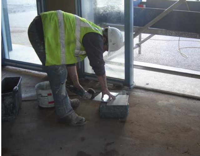
Cutting ceramic wall tiles
