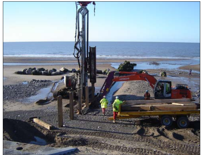
Driving the greenheart timber piles
