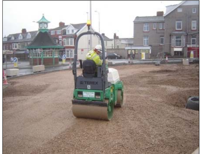
Preparing the plaza area for concreting works
