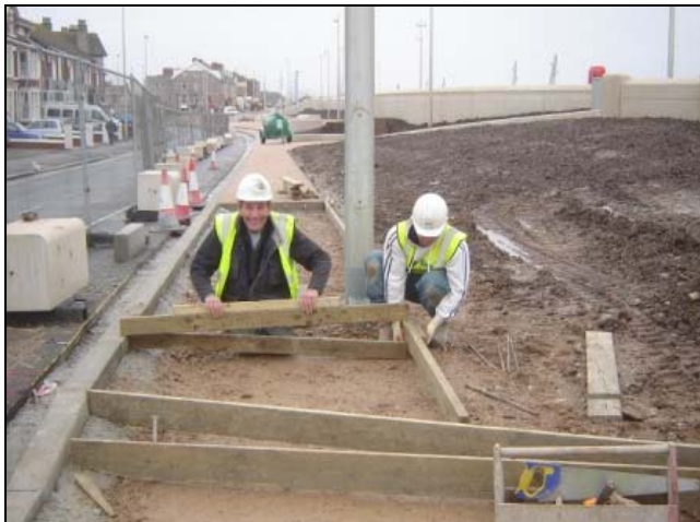
Installation of timber shuttering for new roadside footpath
