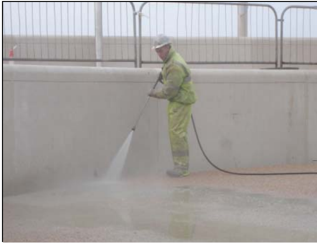
The exposed aggregate finish is revealed by power washing
