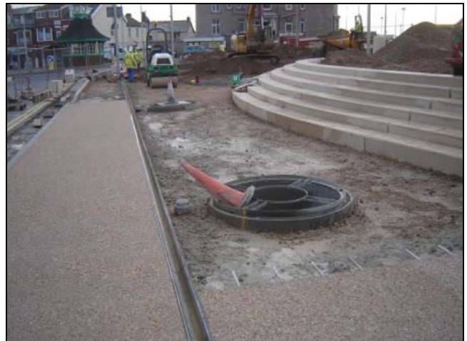
Planters have been installed in the lower plaza
