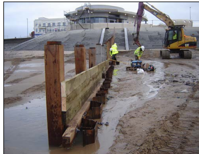
Building the new groynes
