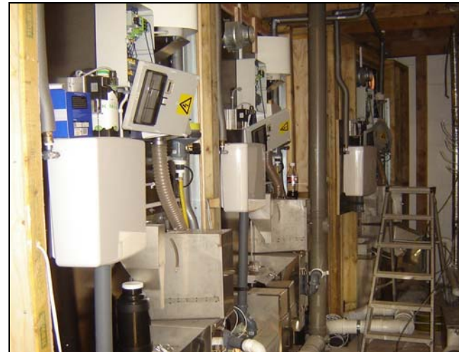
Installation of the toilet facilities – viewed from inside
