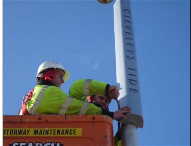
Installation of the illuminated tidal gauge
