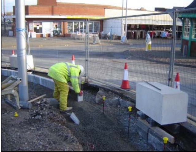
Relining the new kerb alongside South Promenade
