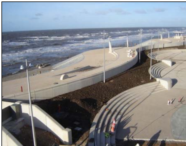
Landscaping works behind seawall
