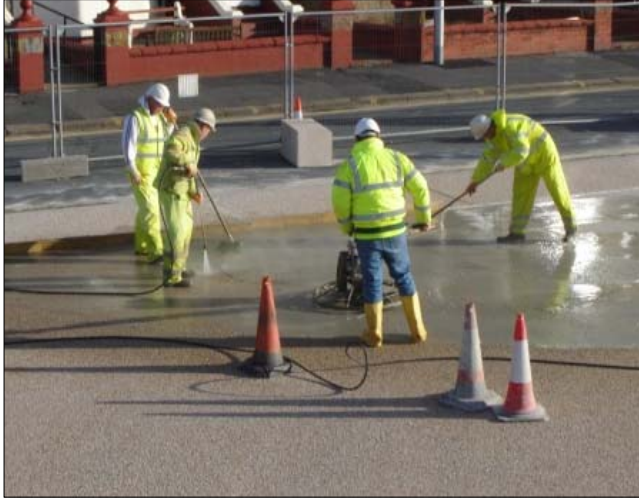
Exposing the coloured aggregate
