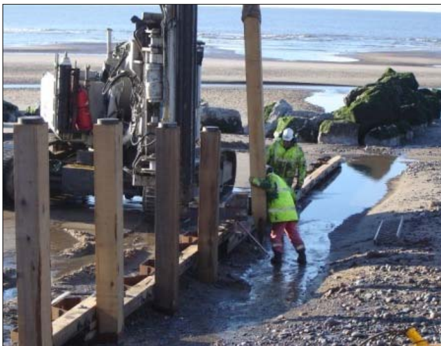
Installing the hardwood timber groyne posts
