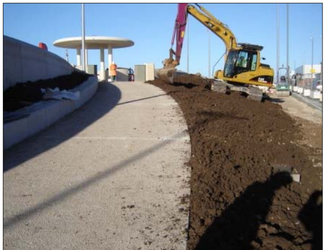
Landscaping works behind the new seawall
