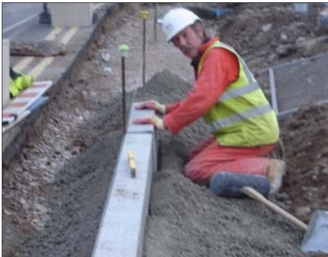
Installing the roadside kerbing
