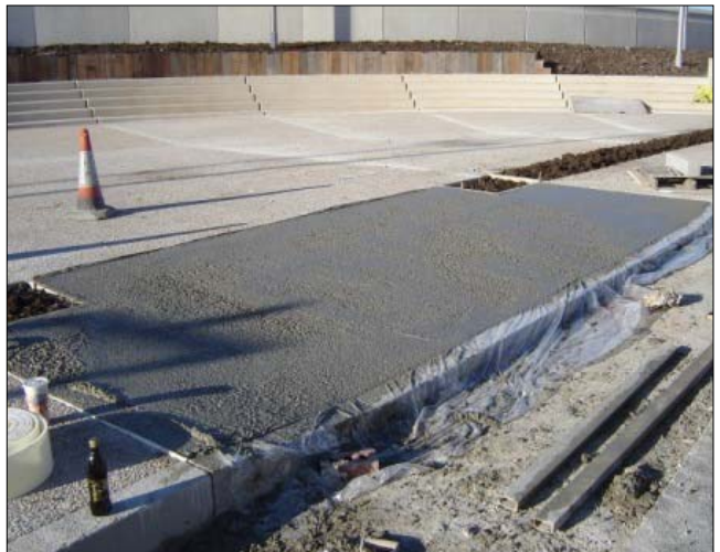
Construction of the roadside pavement
