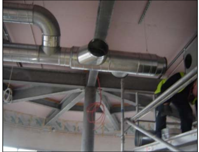
Installing ventilation ducting
