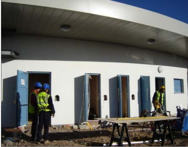
Installation of the toilets has begun
