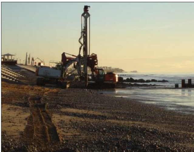
Driving the sheet steel piles into the beach
