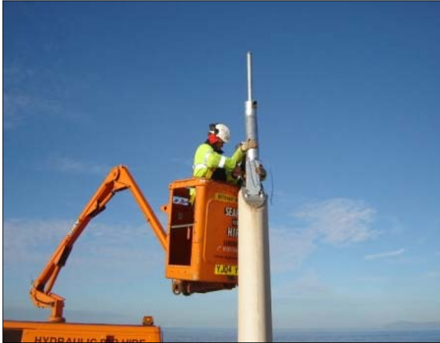
Installation of the new lighting heads
