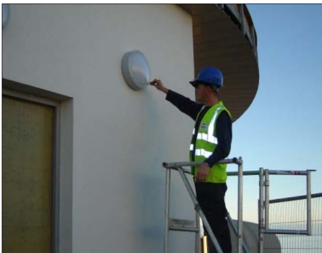
External lighting has been installed to the café
