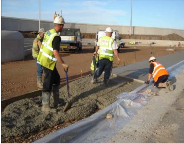
Concreting of the roadside footpath
