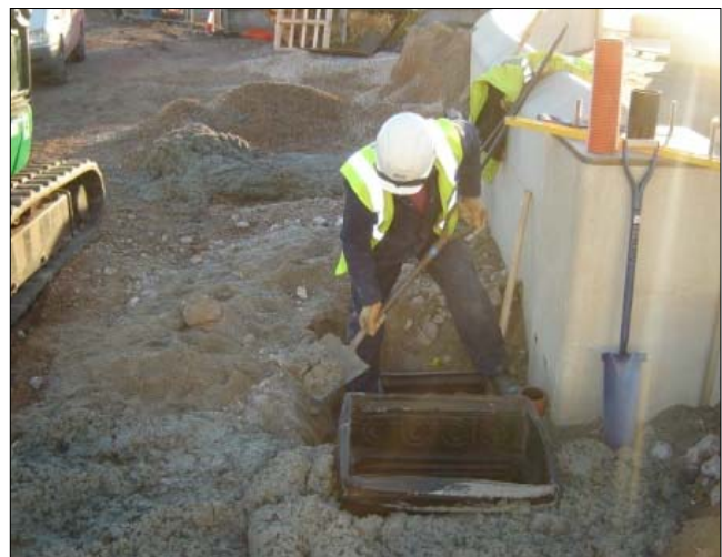
Installing ducting for the wind turbine units
