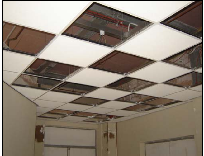
New suspended ceiling in café under construction
