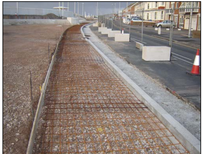
Preparation of the roadside kerbing
