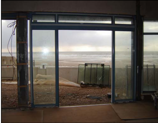
The café windows have now been installed
