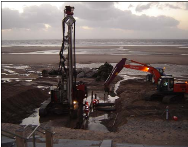
Installation of sheet steel piles in progress
