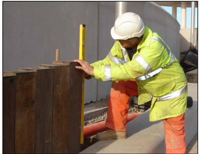
Installing timber retaining wall for landscaping works
