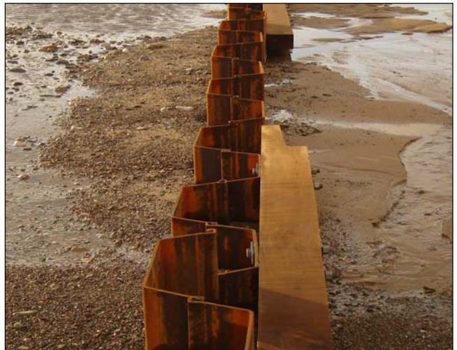
Fixing of timber walings to sheet steel piles
