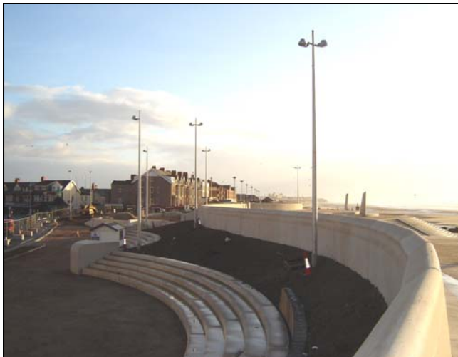
New lighting has been erected in the recreational area
