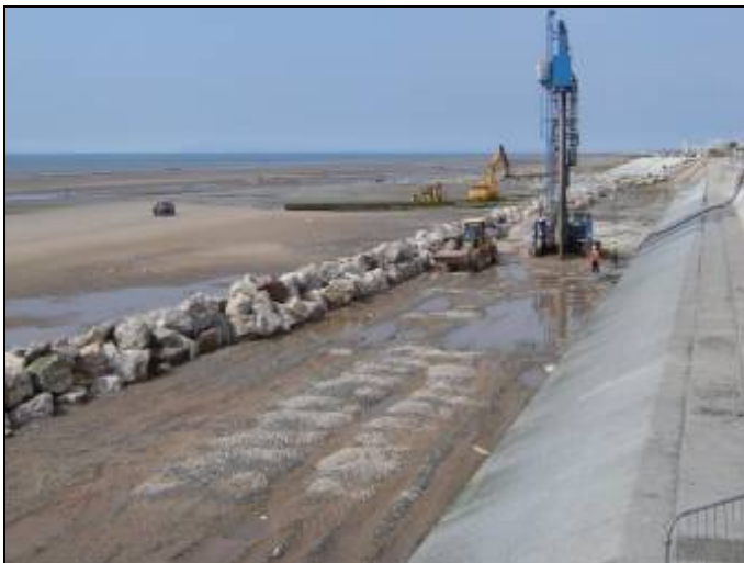
Rock armour being placed on the beach.
