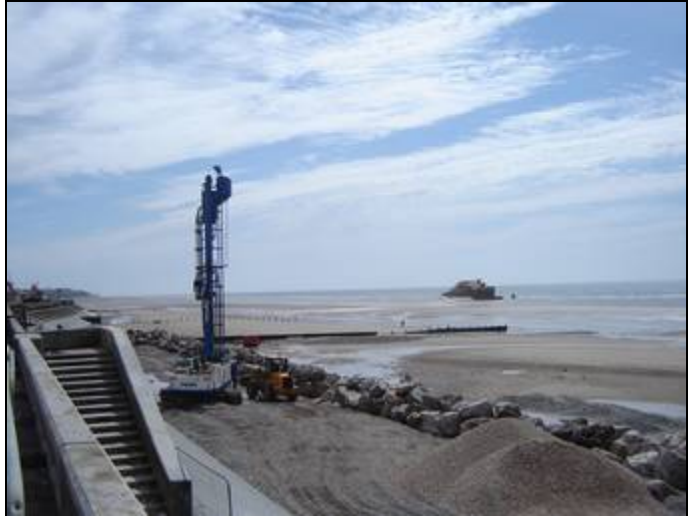
Ground stabilisation works in progress.
