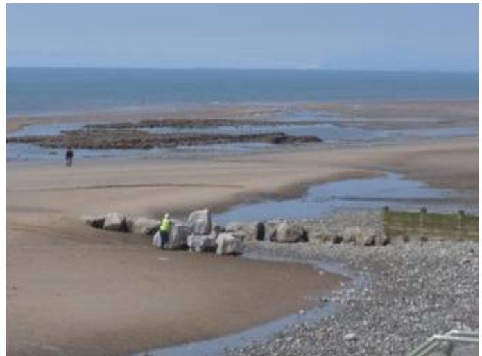
Placing rock armour to extend groynes
