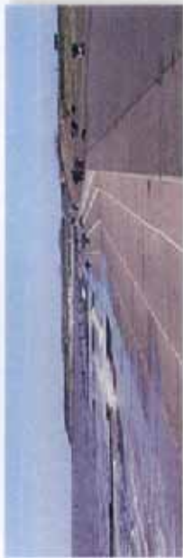
OPTION 3 - LOW WALL WITH STEPPED REVEMENT
